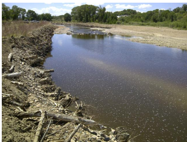
Toe-wood and Rock Vane Structures
